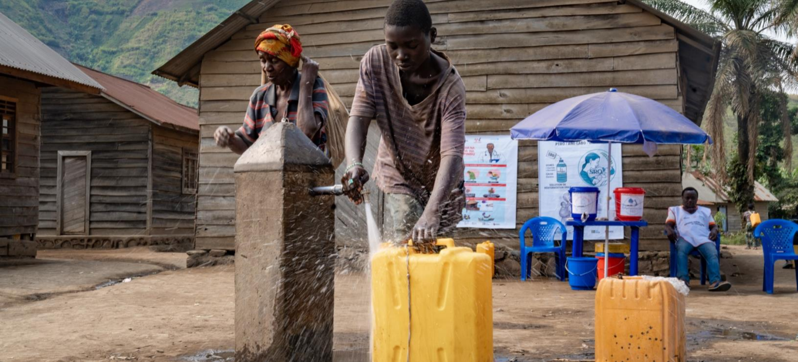
Masisi, Nord-Kivu, DRC. 27 June 2025. A water point constructed by partners and funded by CERF and DRC HF to combat the cholera outbreak in Masisi. Credit: UNOCHA/Wassy Kambale.
