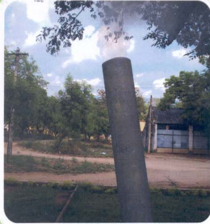
Smoke from the Vent pipe Which is 4 meter above the ground level
