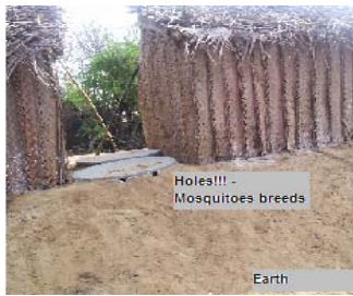
Figure 31 Raised Pit at Tharangampadi, Tsunami affected village, Tamil Nadu
