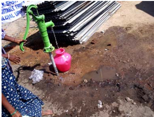
Figures A Shallow hand pump – an emergency measure! Quality monitoring is a regular one!!! (Platform with lead to a drain for spilled water are missing).
