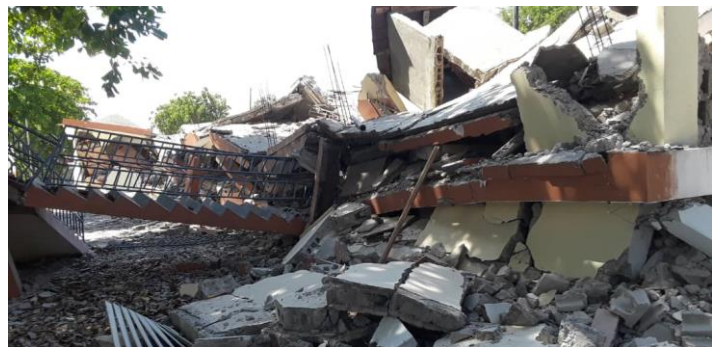
Collapsed buildings in Jérémie. Source: IFRC, 14 August 2021.
