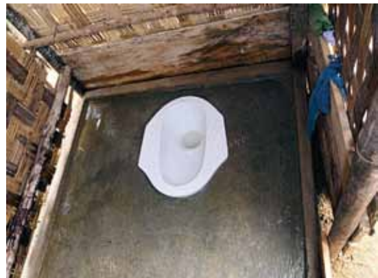
In many Asian countries, like the above example from Vietnam, the pour-flush toilet with off-set tank is the preferred sanitation option
