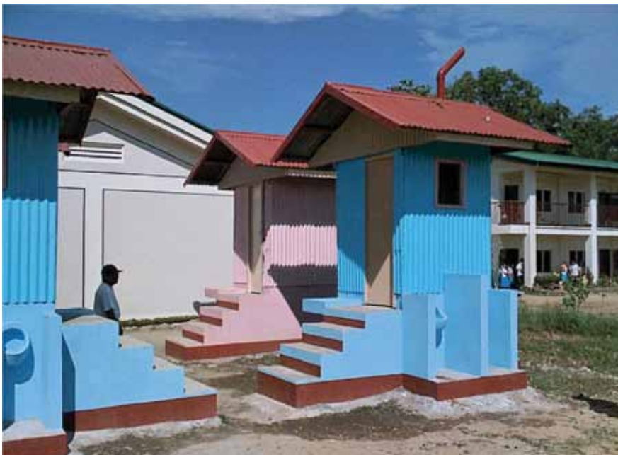
Double-chamber school UDDTs in Negros Oriental, Philippines (source: Robert Gensch 2009)
