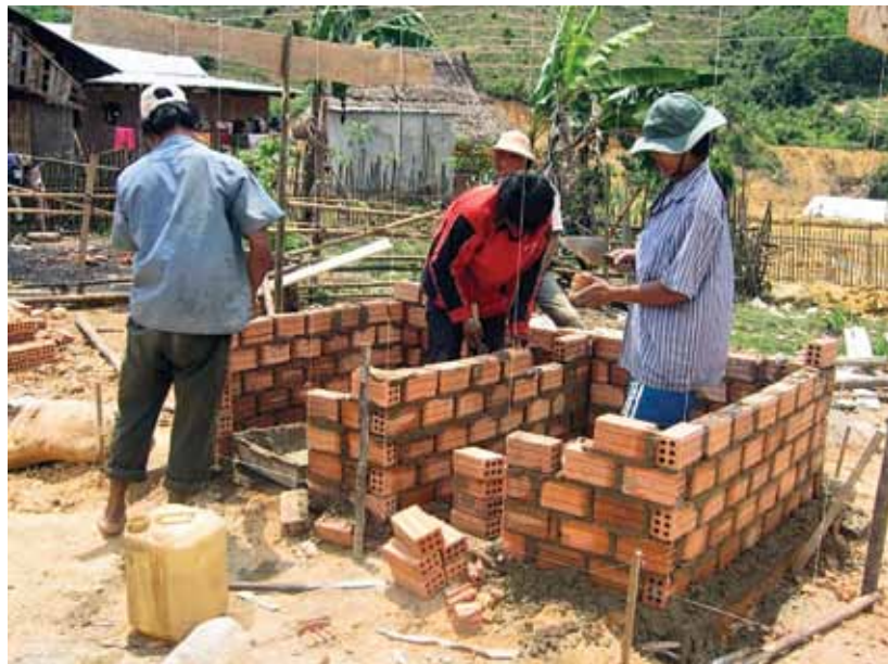
Latrine construction in Vietnam
