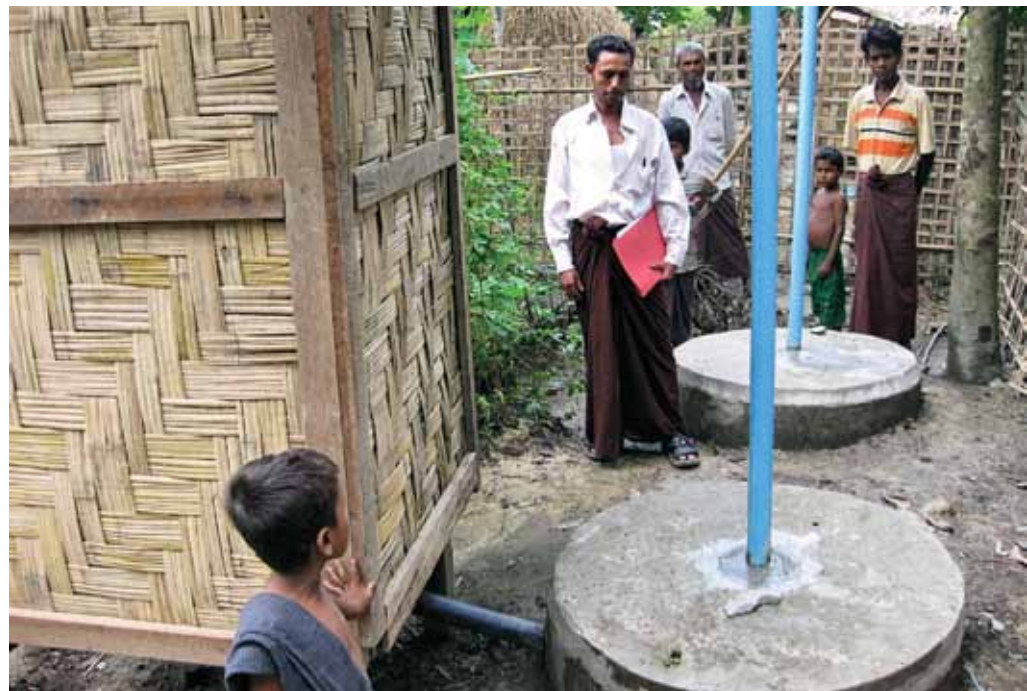
Double Pit Composting Latrine, Myanmar
