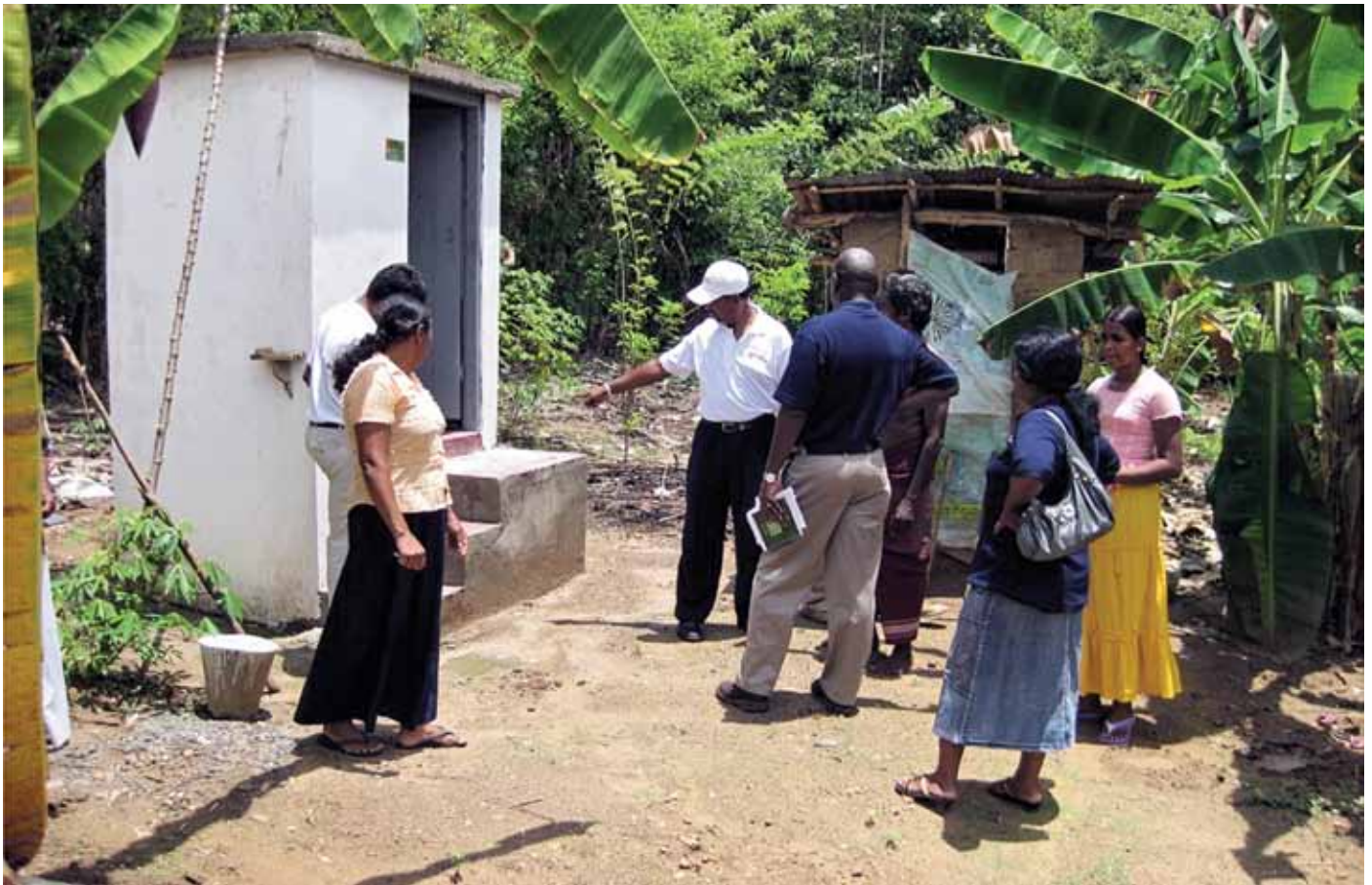
Dry composting eco san latrine in Dehiathakandya, Sri Lanka
