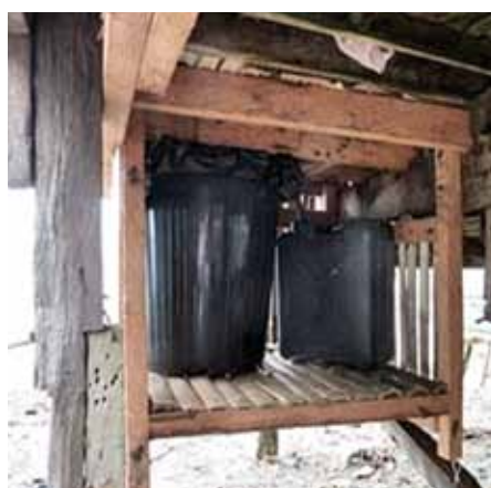
Hanging UDDT examples in a coastal fisher community, Mindanao, Philippines (Source: Gensch 2008-10)
