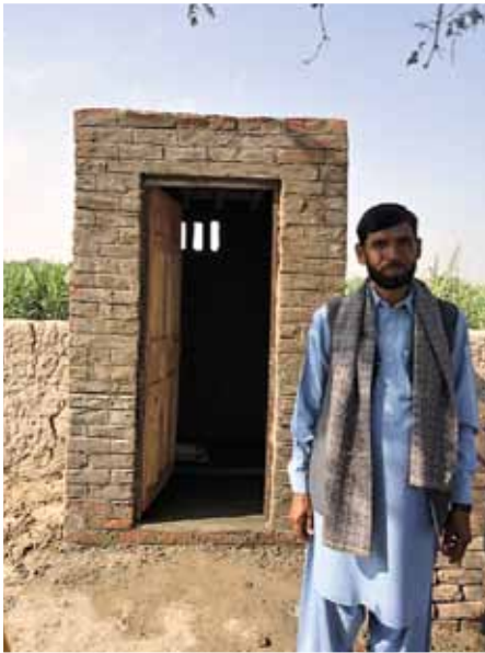
Latrine construction, Pakistan
