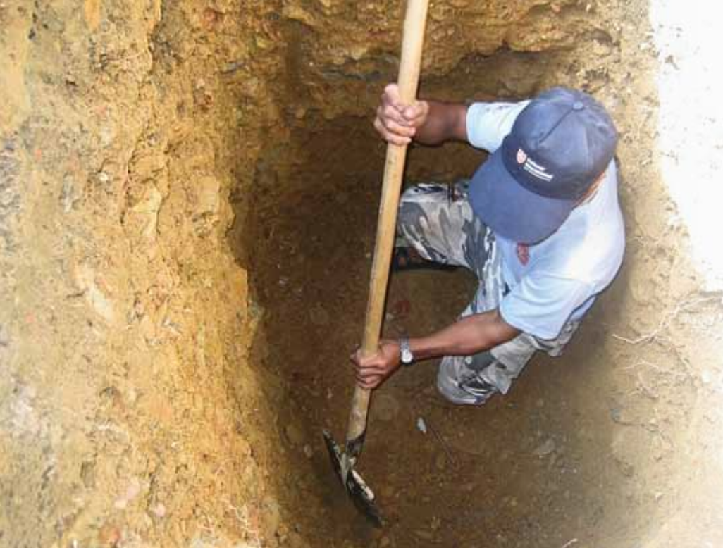
Latrine pit digging, Vietnam
