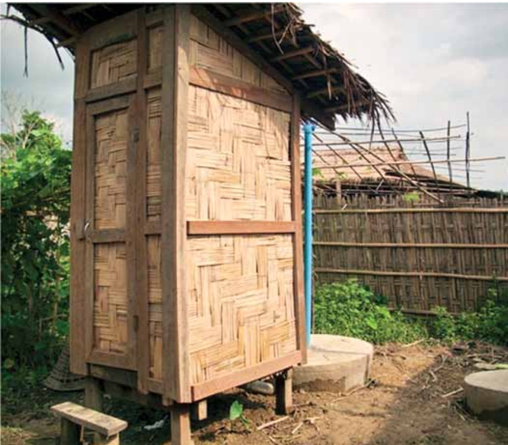
Double pit latrine in NRS, Myanmar. When one pit is full, the contents will be covered with soil for composting (about 18 months) and the superstructure will be lifted up and positioned for use with the second pit. This idea of a "mobile superstructure" came from the villagers themselves.
