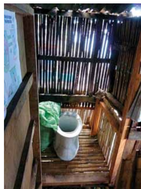
Hanging UDDT examples in a coastal fisher community, Mindanao, Philippines (Source: Gensch 2008-10)
