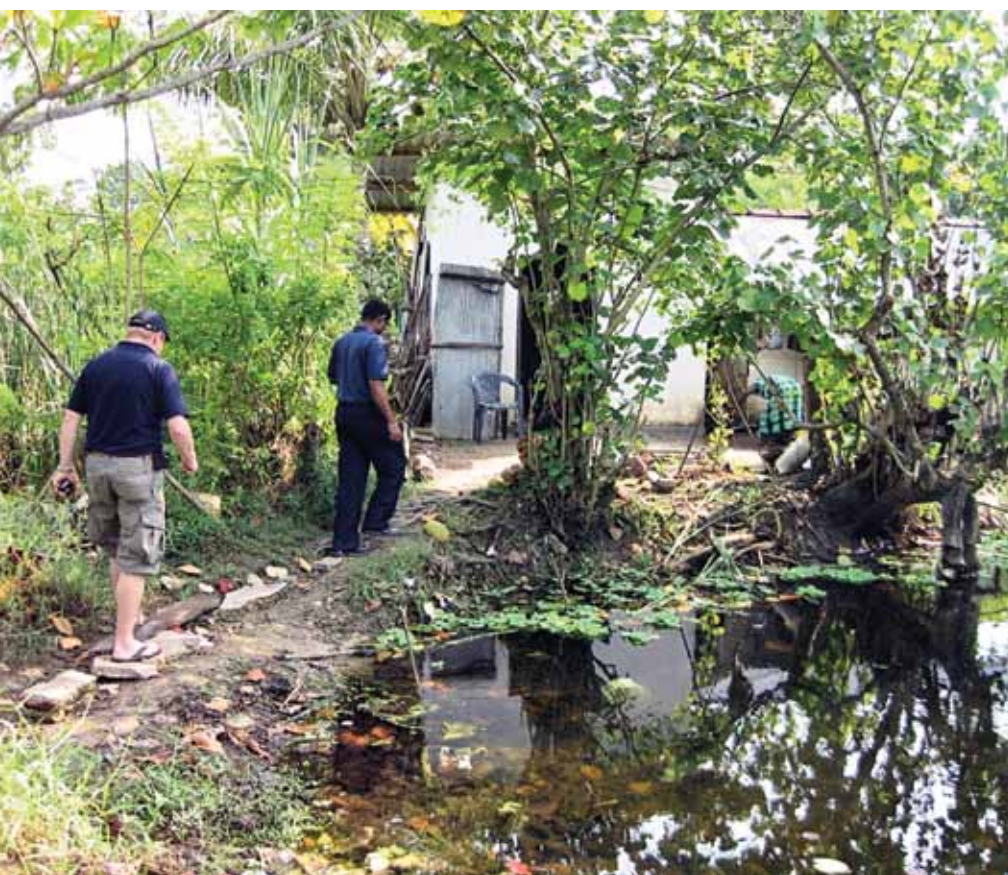
In areas with high water tables, like here in Habaraduwa, Sri Lanka, dry compost raised Ecosan latrines are often one of the few options possible
