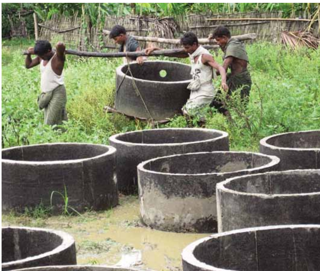
Concrete ring manufacturing in Buthidaug, Myanmar
