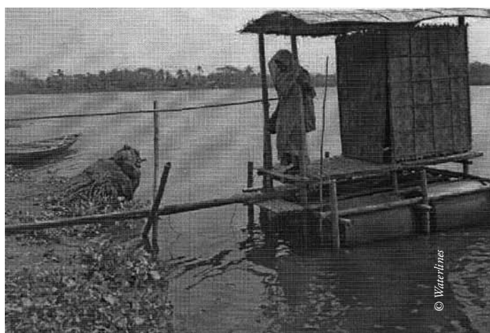
The floating latrine may be used where there is no space on dry land to build a toilet
