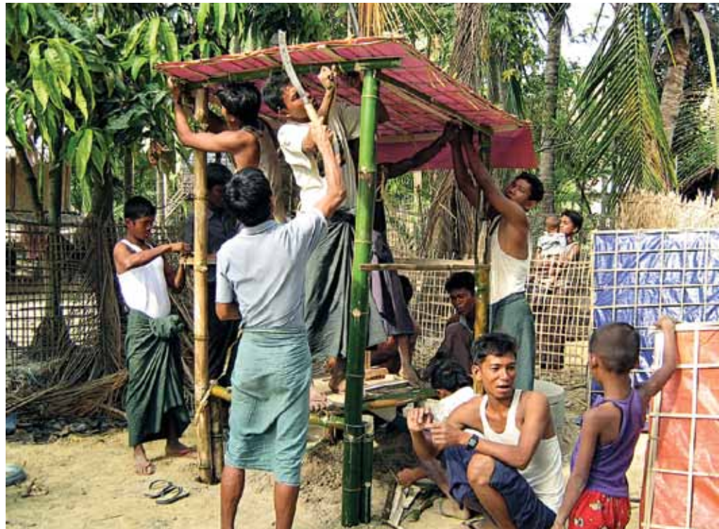
Latrine construction, Myanmar
