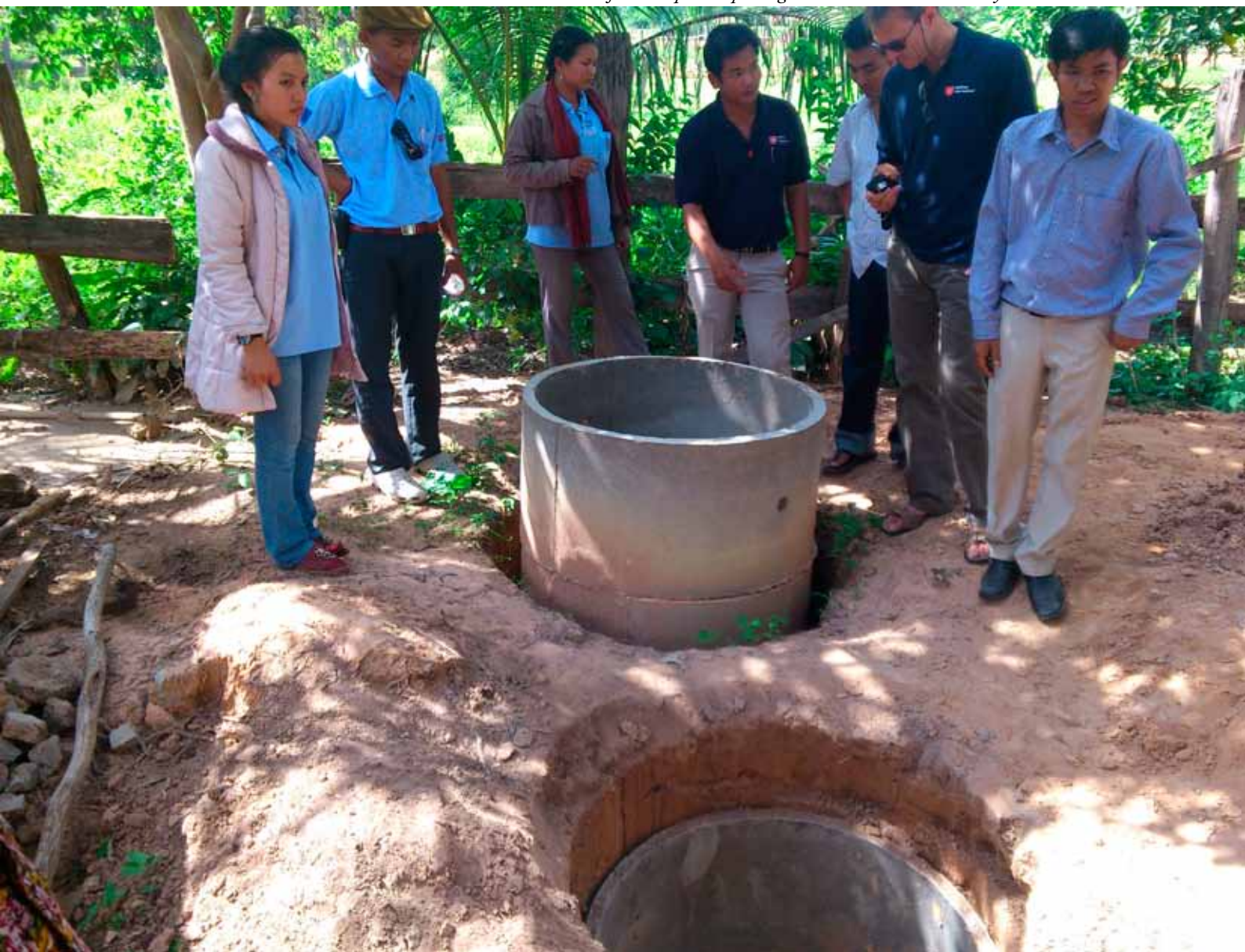
Installation of double pit composting latrine in Oddar Meanchey Province, Cambodia.
