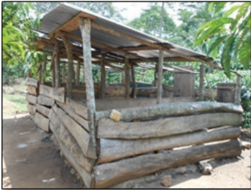
Figure 8. House made of timber walls and iron roof.
