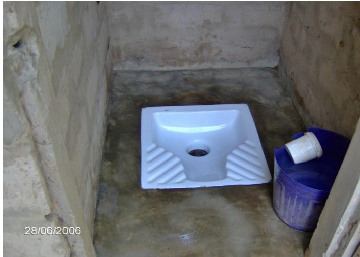
Interior of Manual Flush Latrine
