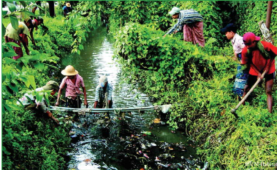
Clearing drainage by the community
