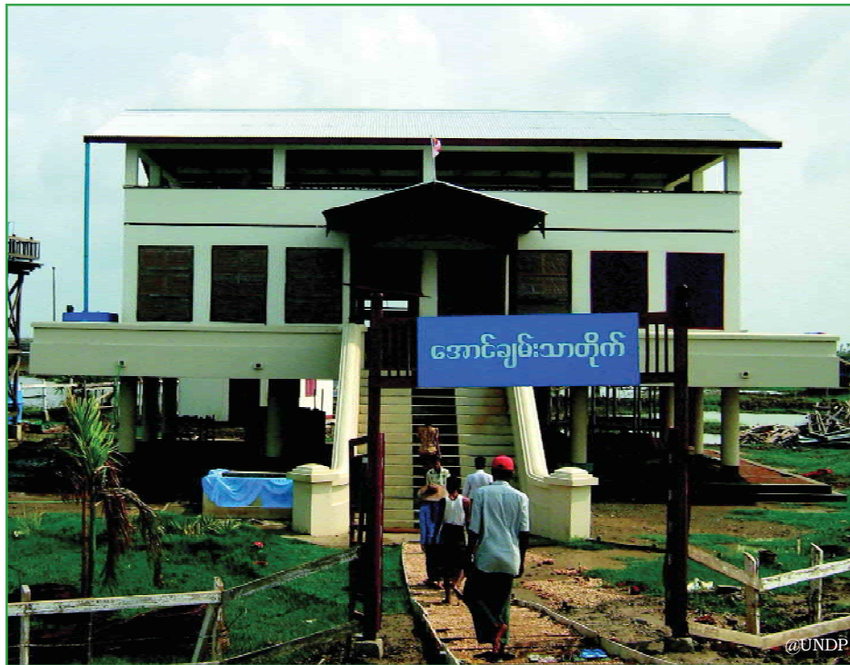
A monastery elevated on posts, piles above flood level so that the community can use it as a shelter during a flood.
