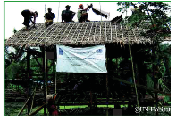
A training for carpenters to enhance community-based disaster mitigation
