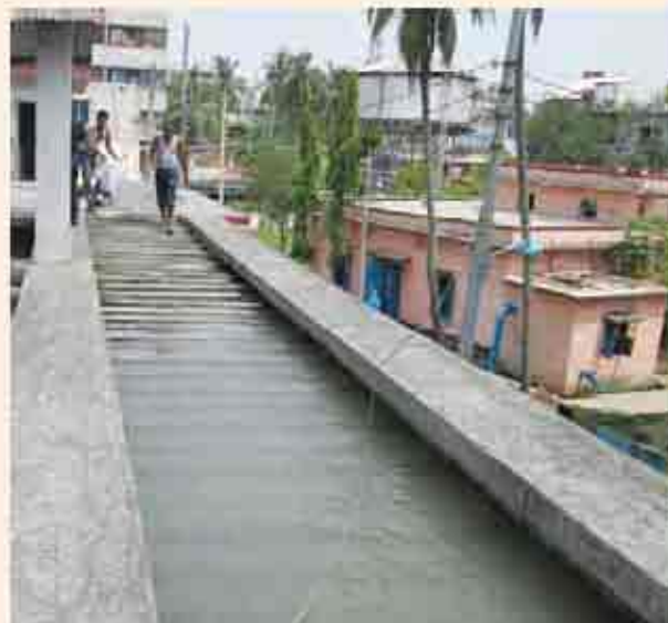
4. Promoting flocculation in baffle channel
