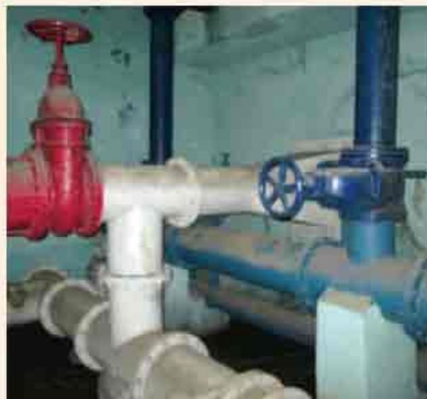
2. Water lifting through pump
