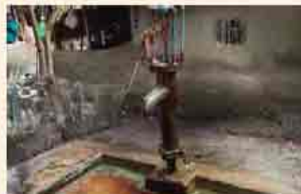
Lid on the top of the pump
