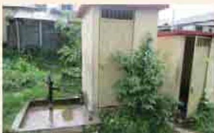
Latrines less than 30 feet from tubewell
