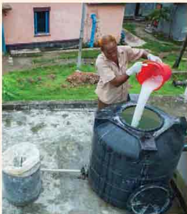
7. Disinfection (with chlorine) to kill microorganisms
