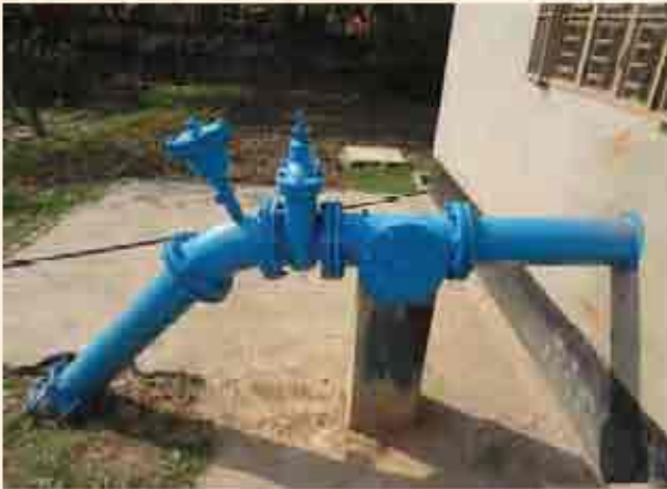
10. Groundwater is lifted by pump
