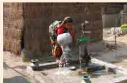
Sanitary seal exists and cloth/bottle is not fastened at the mouth of the pump
