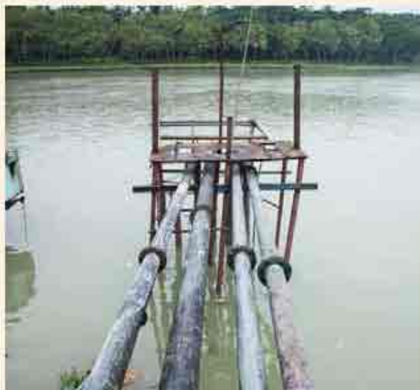
1. Collection from surface water source through intake
