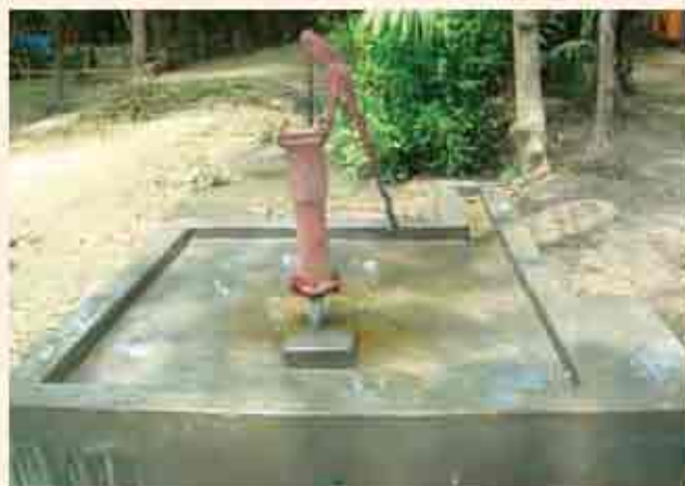
Tubewell technology which uses groundwater
