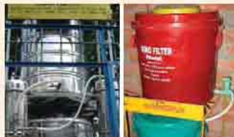
Arsenic and/or iron removal filters/plants
