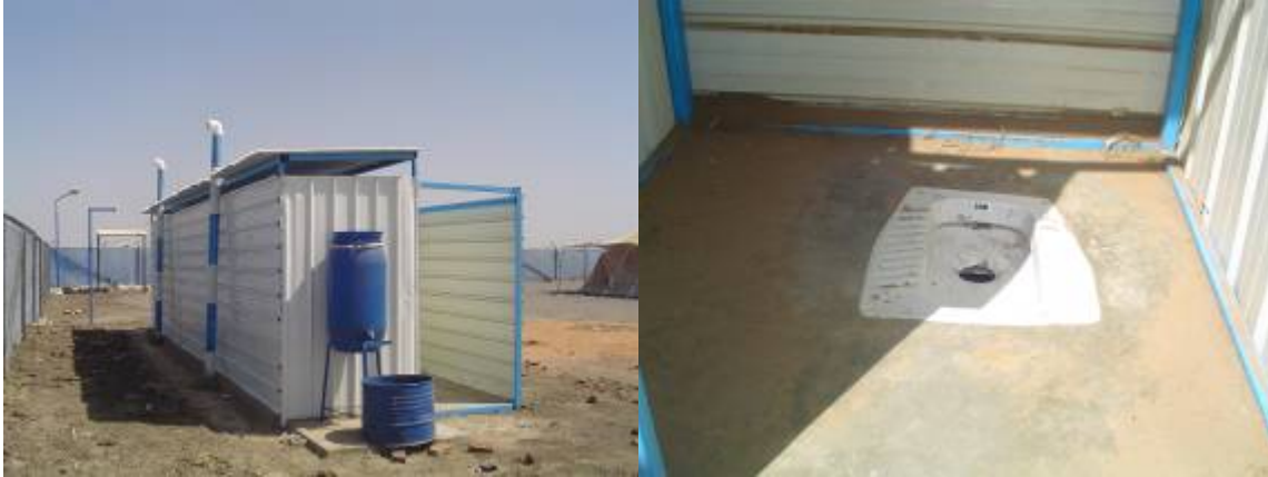
Figure 8: Superstructure of a latrine made from corrugated iron sheet and RHS
