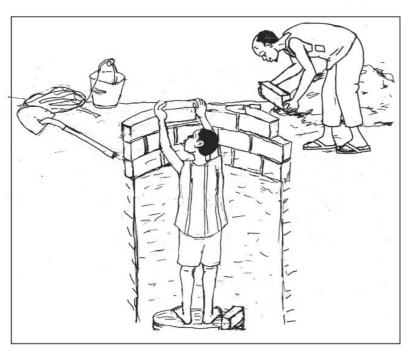
Whatever type of soil you have, the sub foundation at the top 50 cm of the pit must be lined with concrete bricks or with rubble stones.
