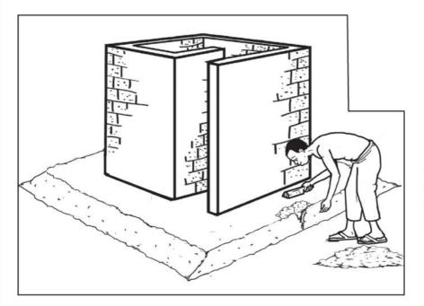
You have to maintain the latrine regularly: fill holes made by rodents, frequently patch the embankment around the latrine, maintain the superstructure, etc.
