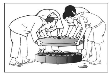
You must earth up the soil around the sub foundation to avoid stagnant water accumulating around the latrine.
